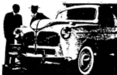
Here is the auto Henry Ford "grew from the soil." Its plastic panels, with impact strength 10 times greater than steel, were made from flax, wheat, hemp, spruce pulp
